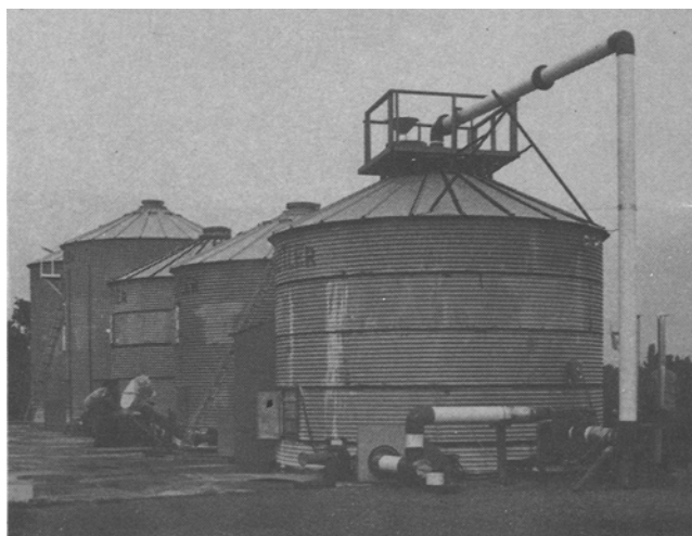
FIG. 1. Actual bin used in the application of ammonia and for recirculation of the air to ensure uniform distribution of moisture and ammonia in the corn during the detoxification process.
